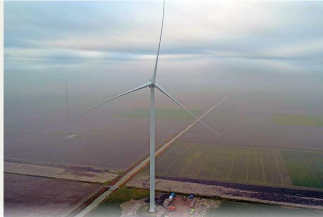
Special feature... GE's 5.3MW Cypress prototype in the Netherlands has segmented blades
